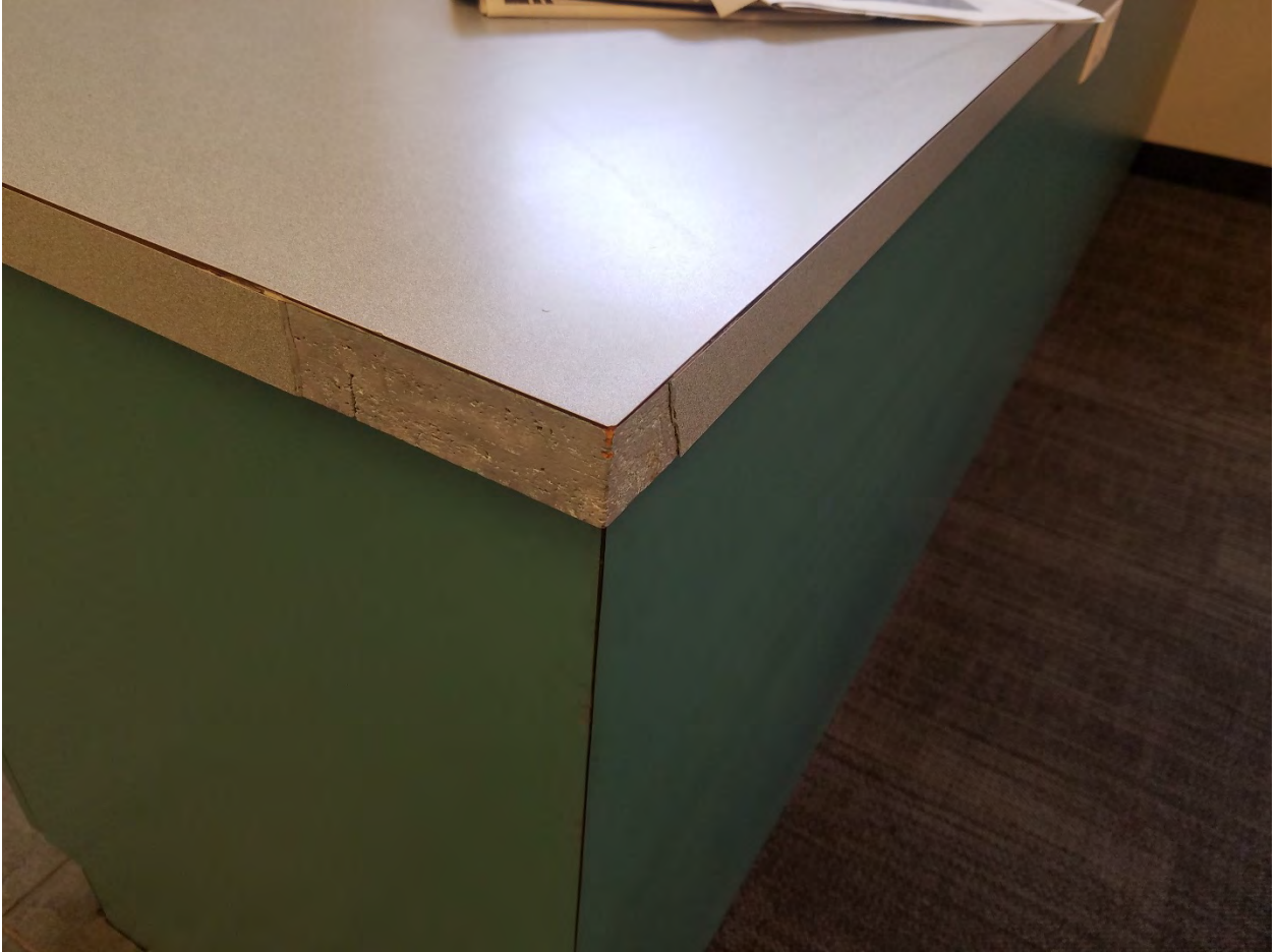
Missing laminate corner on counter in Staff Lounge
