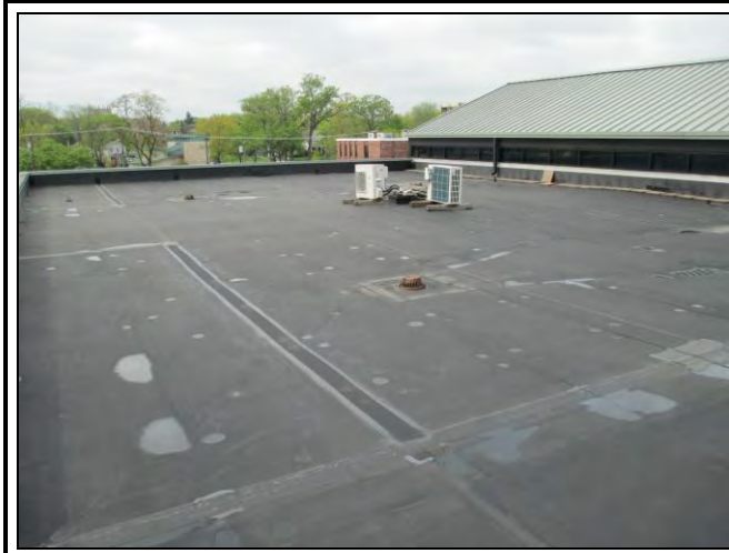
Photo 3: Roof Area 3: Looking south across the fully adhered EPDM roof cover of area 3, within the inside of mechanical screen wall.
