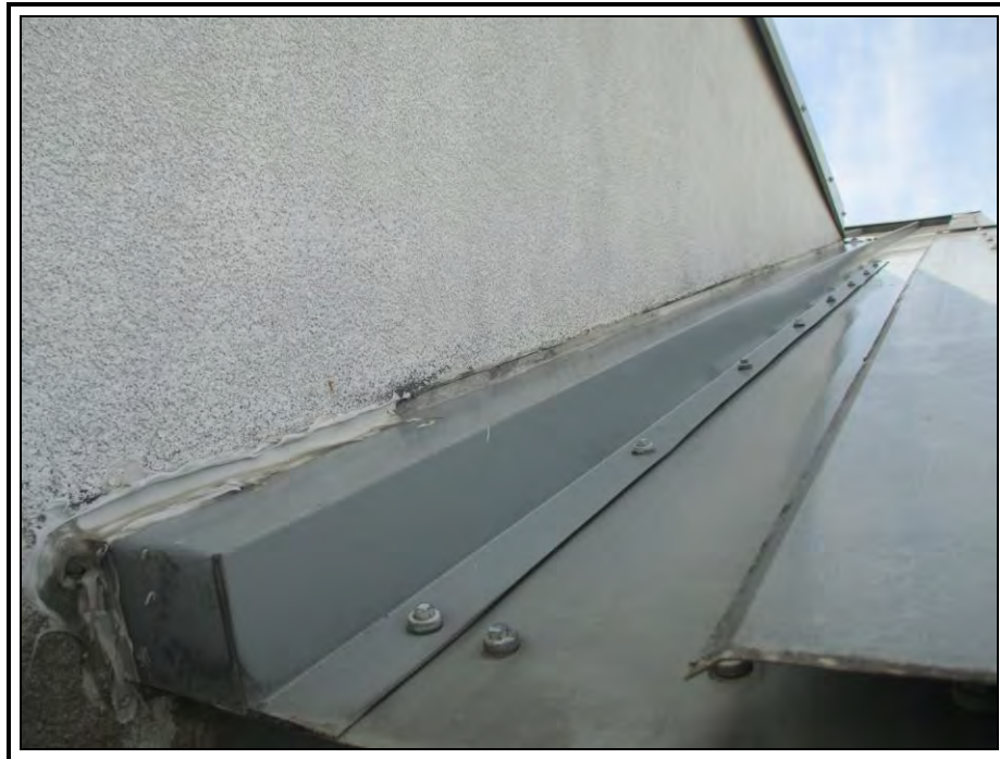
Photo 31: Roof Area 2 and 4: The EIFS mechanical screen wall intersects the south roof rake edges of the standing seam roofs creating a difficult flashing condition. Note the different color sealant, a sign of previous repair.
