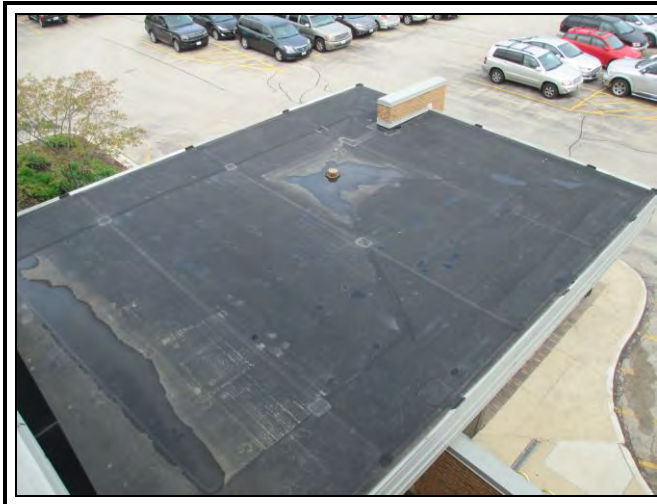
Photo 1: Looking down at Roof Area 1: Fully Adhered EPDM.
