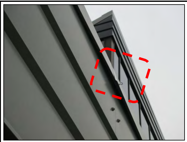
Photo 21: The east roof edge coping on roof area 1 is partially disengaged from the clip and should be reset.
