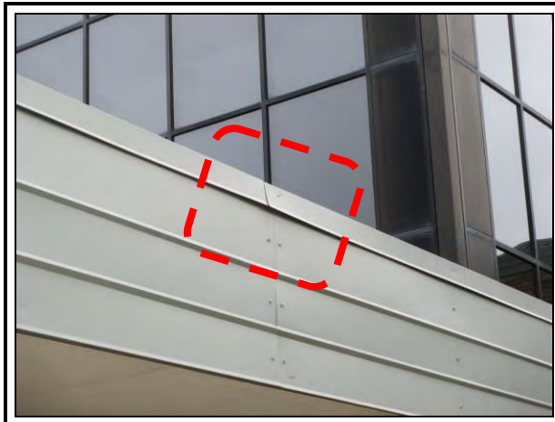
Photo 21: The east roof edge coping on roof area 1 is partially disengaged from the clip and should be reset.
