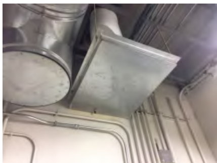
Figure 4: Safe pan not piped to floor drain.
