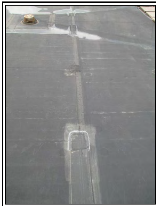
Photo 15: Many of the seams have had cover strips partially installed, apparently due to lack of seam integrity. A way to extend the life of the roof would be to installed 6" cover strips over all of the seams.
