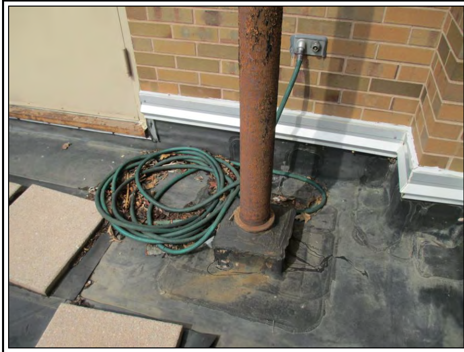
Photo 36: Roof area 9, the pipe penetration in the northwest corner of the roof is flashed with a pourable sealer pocket. At this time the pourable is in fair condition, but should be checked regularly for debonding from the pipe, slumping and the need for additional pourable sealer.
