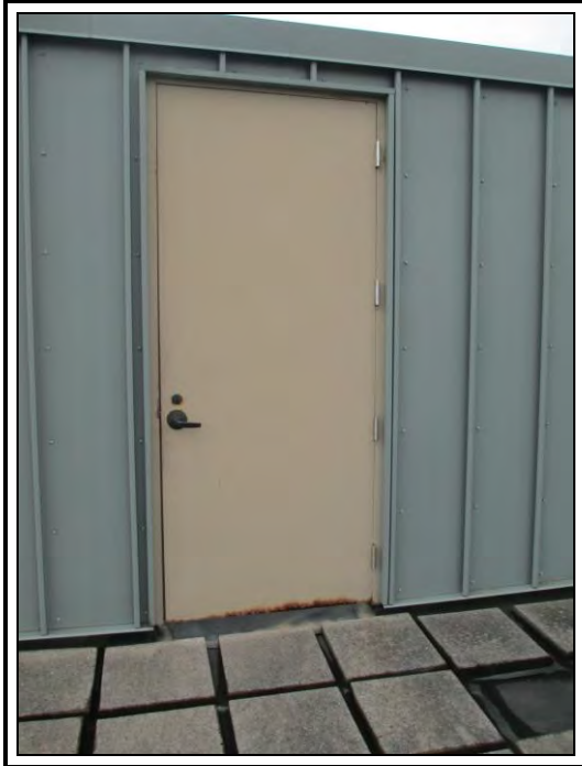
Photo 30: The bottom of the roof top mechanical screen wall door on roof area 3 is beginning to rust.
