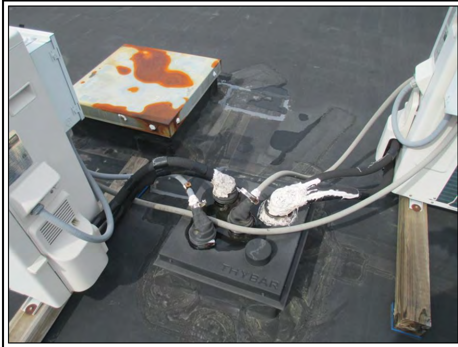
Photo 26: The pipe portal curb has multiple penetrations passing through it. Note the heavy layers of sealant installed at the base of the pipes. This is not a long term solution and a new pre-fabricated pipe penetration house should be installed.
