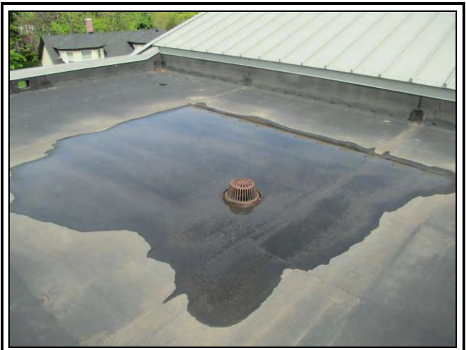
Photo 23: Although it rained the previous evening, large amounts of water were observed ponding around the roof drains on roof areas 3 and 12, respectively.
