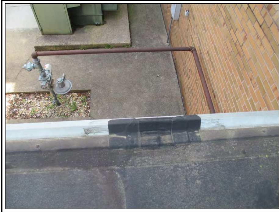
Photo 20: The west roof edge in the southern portion of roof area 1 has been repaired with an EPDM patch.
