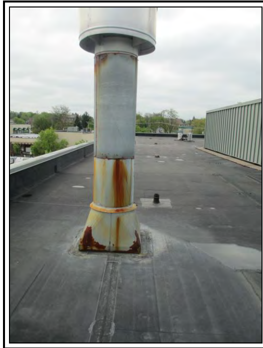
Photo 24: Roof area 3: The square to round flue flashing and flue section is made from galvanized steel and are beginning to rust and should be replaced with a new stainless steel square to round flashing and flue section should be installed.
