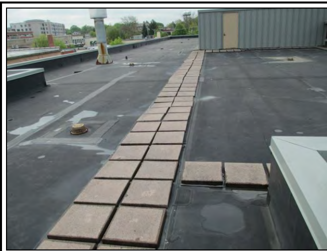
Photo 29: Concrete pavers set on a sacrificial EDPM sheet are spread across roof area 3 and 9.
