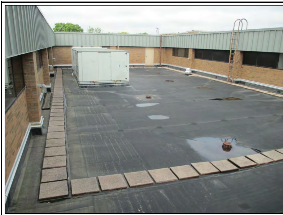
Photo 9: Looking west across Roof Area 9: Fully adhered EPDM.
