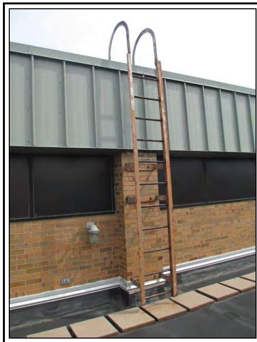
Photo 35: The existing ladder from roof area 9 to 10 is beginning to rust and should be removed and prepped, primed, painted and reinstalled. Additional pavers should be installed below the bottom of the ladder.
