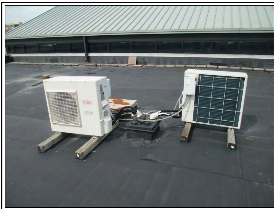
Photo 25: The air conditions have been placed on 4x4 wood blocking rails on bearing pads. The 4x4s are not long term solutions and should be replaced with 2'-0" x 2'-0" x 2" rubber walk way pads.
