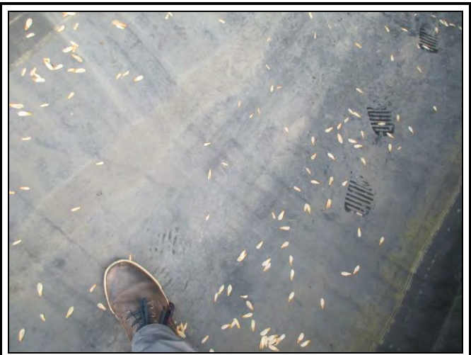
Photo 33: Roof Area 5 and 6: Portions of the EPDM on this area felt unadhered under foot. The loose EPDM and insulation below should be removed and a new installed.
