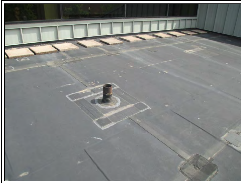
Photo 18: Many of the penetrations across the EPDM roof area have been reflash.
