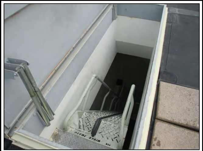
Photo 28: The roof areas are accessed via a ships ladder with offset steps and roof hatch at the north end of roof area 3. The hatch lid is heavy and difficult to open.
