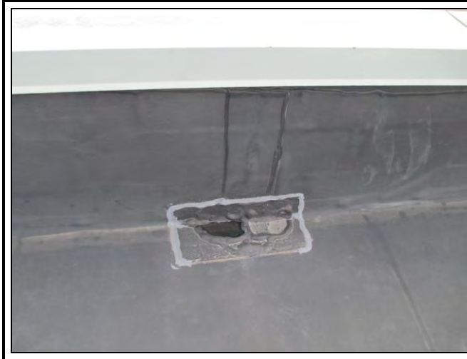
Photo 14: Numerous patches were observed at the angle change between the roof and the parapet wall. The grey color sealant around the perimeter of the patch is polyurethane sealant, typically not used to seal the edges of the EPDM patch. EPDM lap sealant should be installed and tooled over the edge of the patch.
