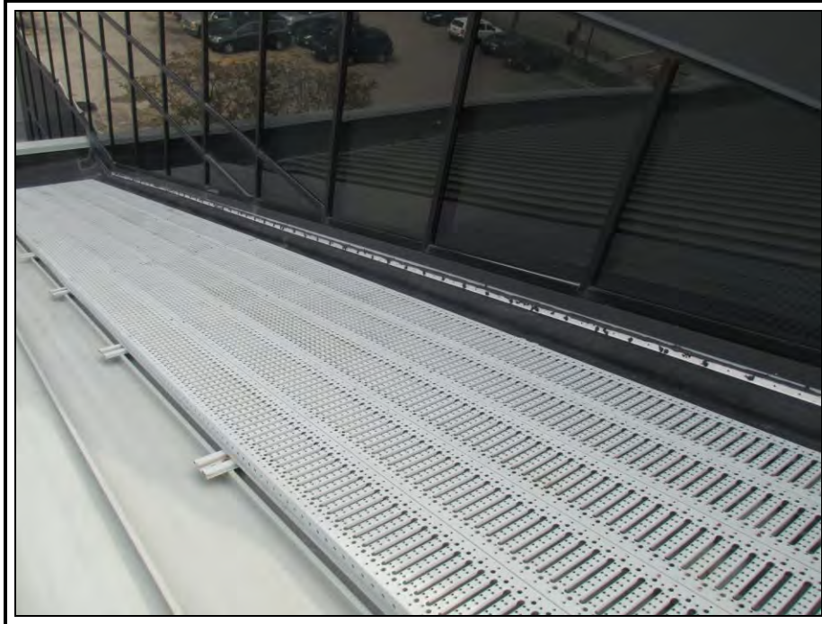
Photo 38: At the east end of roof areas 7 and 10 a walkway grate has been installed over the standing seam roof to ease access to the lower roof areas. Unfortunately, it does not align with the ladder from roof area 9 up to roof area 10 and the standing seam roof needs to be traversed.
