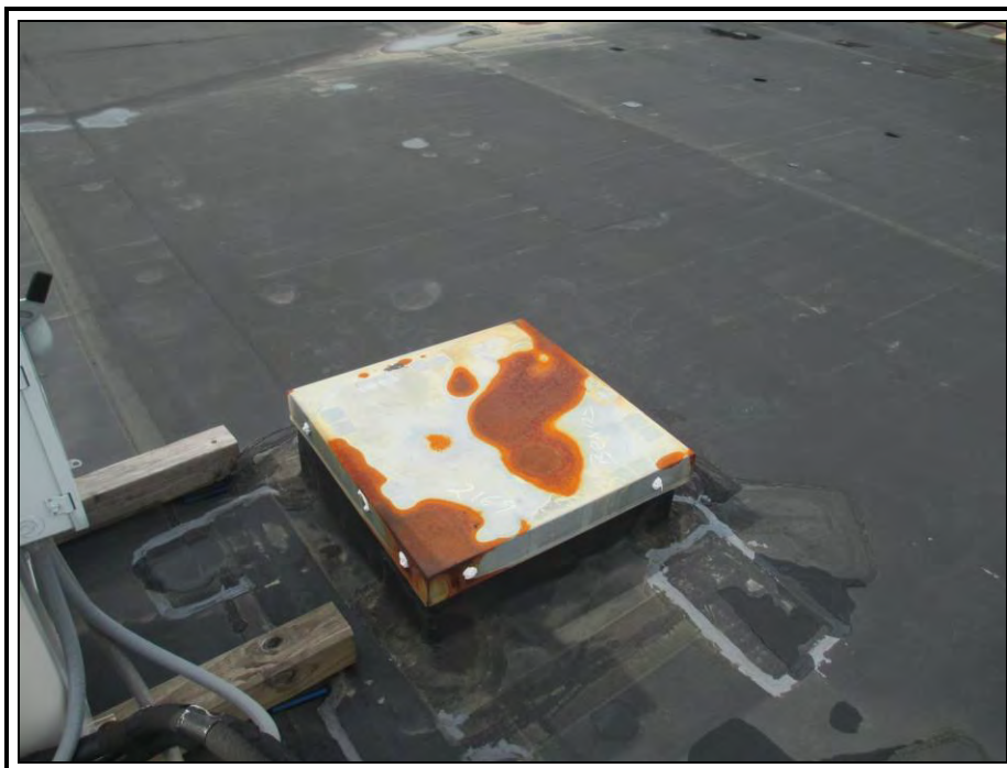
Photo 27: The abandoned roof curb should be removed, new insulation installed to match the height when the roof is replaced in the future.
