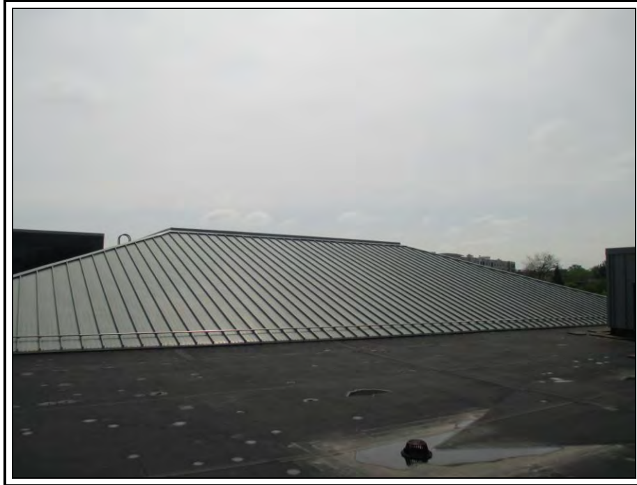
Photo 8: Looking east across Roof Area 8. Prefinished steel standing seam roof.
