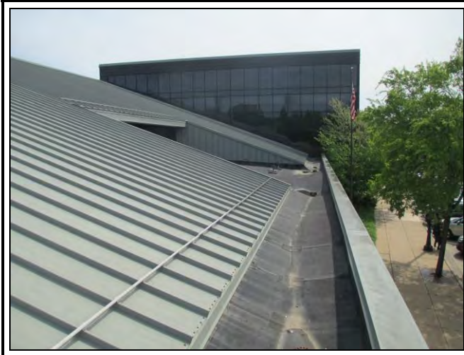
Photo 6: Looking east (left photo) across the prefinished steel standing seam roof and north (right photo) across the fully adhered EPDM section within Roof Area 6.
