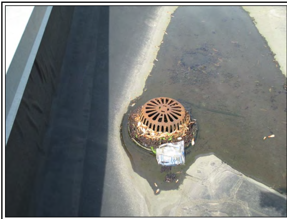
Photo 17: All Roof drains: All debris, both organic and trash should be removed from the roof drain domes.
