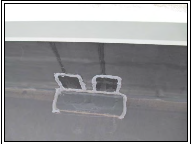
Photo 14: Numerous patches were observed at the angle change between the roof and the parapet wall. The grey color sealant around the perimeter of the patch is polyurethane sealant, typically not used to seal the edges of the EPDM patch. EPDM lap sealant should be installed and tooled over the edge of the patch.
