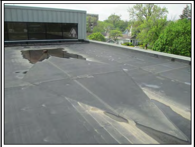
Photo 12: Looking west and south across Roof Area 12: Fully adhered EPDM.
