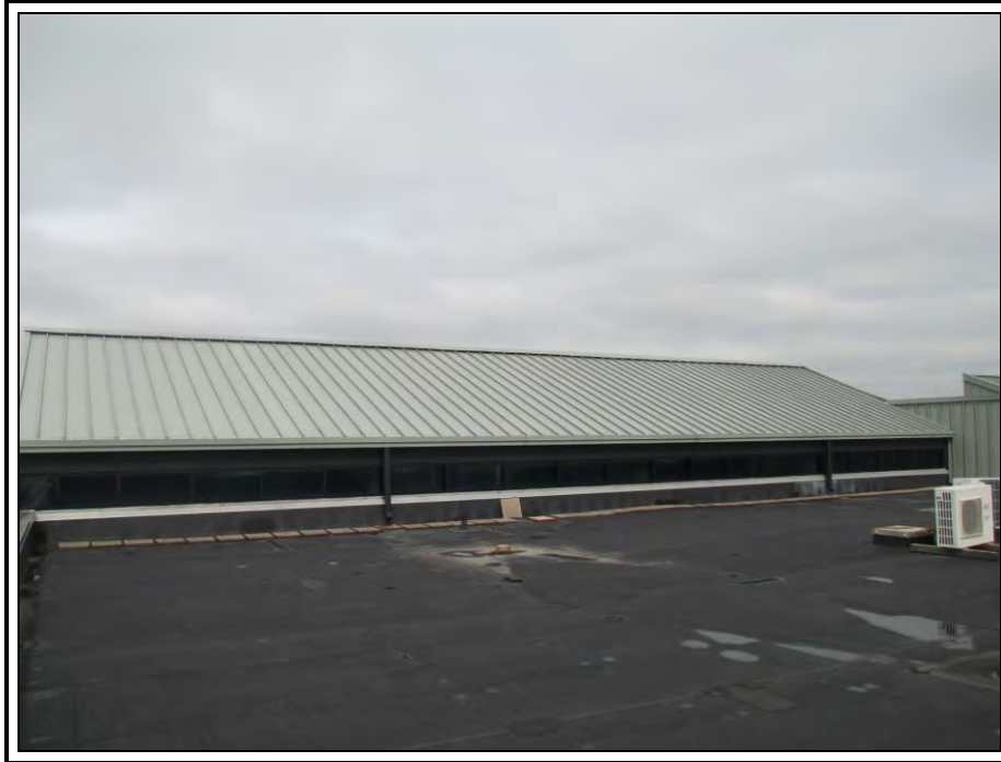
Photo 4: Looking west at Roof Area 4: Fully adhered EPDM.
