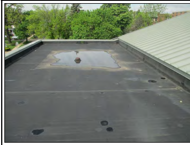
Photo 12: Looking west and south across Roof Area 12: Fully adhered EPDM.
