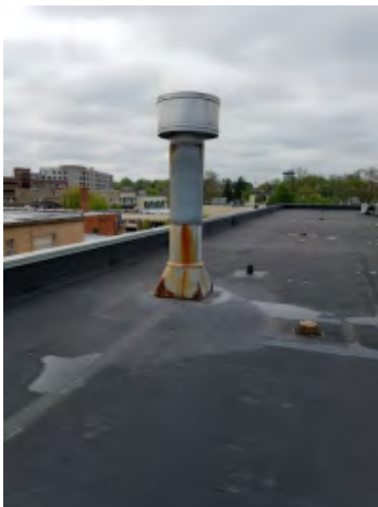
Figure 3: Deteriorating Boiler Flue
