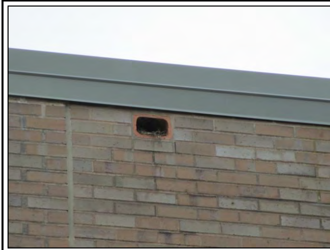
Photo 34: At the west end of roof areas 11 and 6 respectively, the sheet metal scupper framing is missing.
