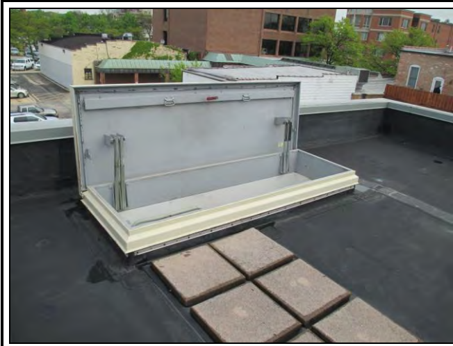
Photo 28: The roof areas are accessed via a ships ladder with offset steps and roof hatch at the north end of roof area 3. The hatch lid is heavy and difficult to open.
