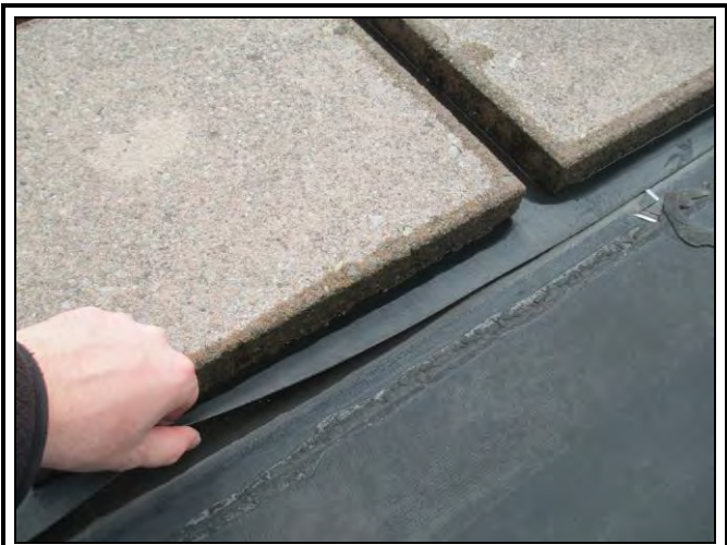
Photo 29: Concrete pavers set on a sacrificial EDPM sheet are spread across roof area 3 and 9.
