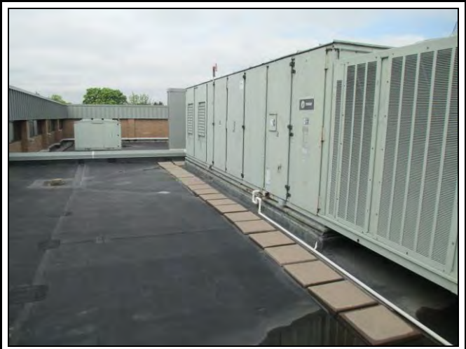
Photo 3: Roof Area 3: Looking south across the fully adhered EPDM roof cover of area 3, within the inside of mechanical screen wall.
