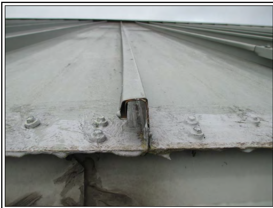
Photo 37: The standing seam roofs, roof areas 2, 4, 7, 8, and 10, are single locked that are 2" high and 16" on center. Roof areas 2 and 4 have gutters at the eave with 2 downspouts that drain onto the adjacent roof below. Repair attempts have been made to eave with a coating material.
