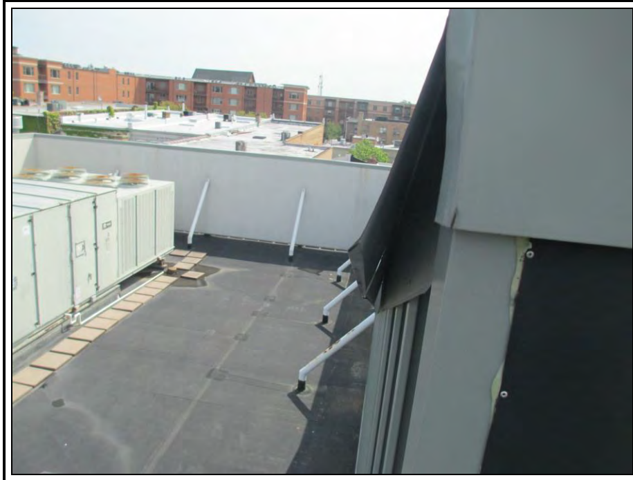
Photo 32: Roof Area 4: The north rake edge of the sheet metal has been disengaged from the clip due to what is presumed to be wind damage. This condition should be repaired as soon as possible to prevent it from blowing off the building.
