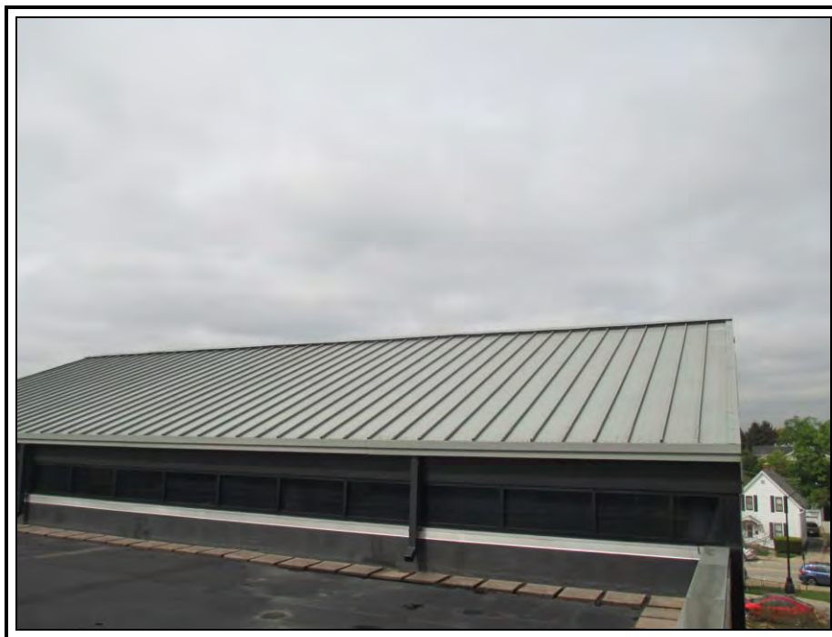
Photo 2: Looking west at Roof Area 2: Prefinished Steel Standing Seam Roof.
