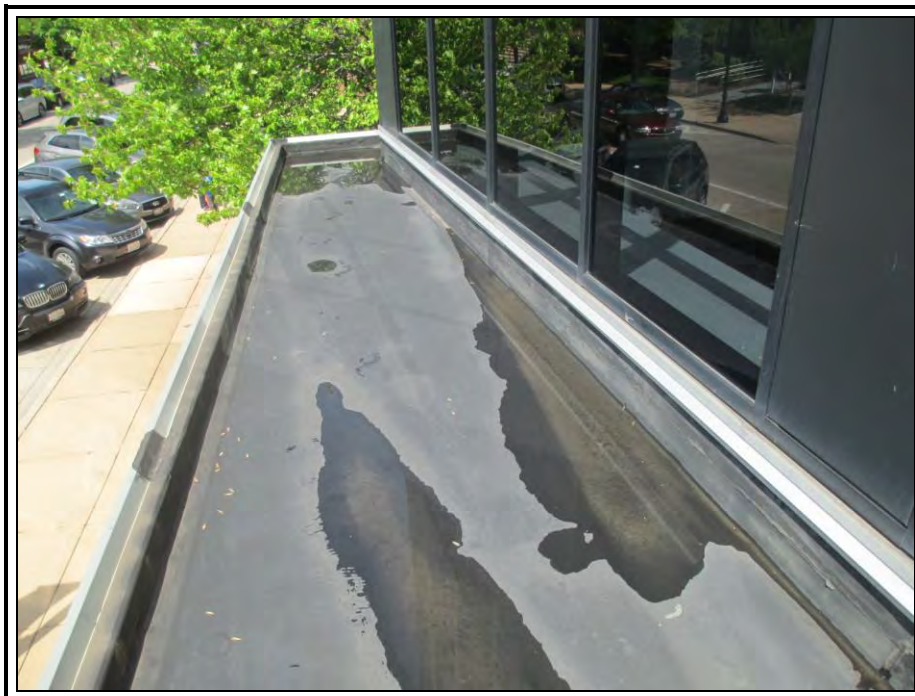
Photo 5: Looking west at Roof Area 5: Fully adhered EPDM.
