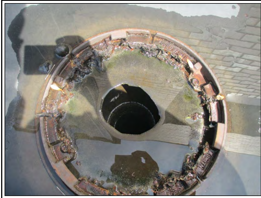
Photo 16: All Roof Areas with EPDM: For the roof drain to function properly the EPDM should be cut back to within ½" of the clamping ring. Here the EPDM restricts drainage.
