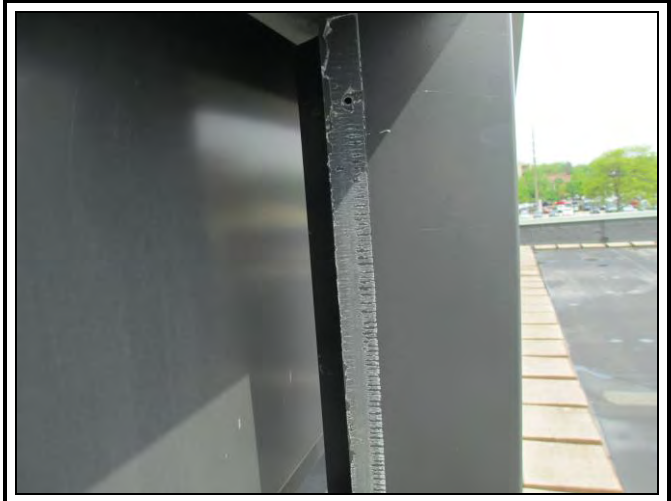
Photo 22: Roof Area 2: The downspout fastener to the outlet pipe is barely secured and needs to be refastened. The fastener holding the downspout together has failed and downspout is open along the back edge.
