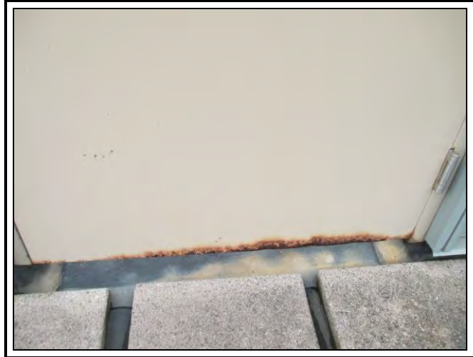
Photo 30: The bottom of the roof top mechanical screen wall door on roof area 3 is beginning to rust.
