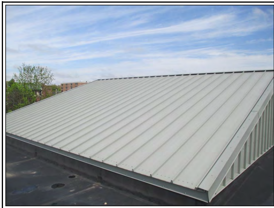
Photo 13: Looking north across Roof Area 13: Prefinished steel standing seam roof.
