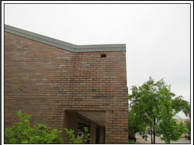
Photo 34: At the west end of roof areas 11 and 6 respectively, the sheet metal scupper framing is missing.
