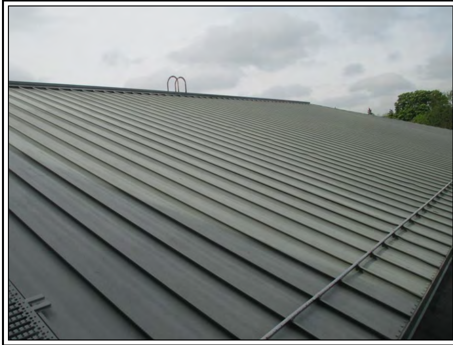
Photo 10: Looking south across Roof Area 10: Prefinished steel standing seam roof.
