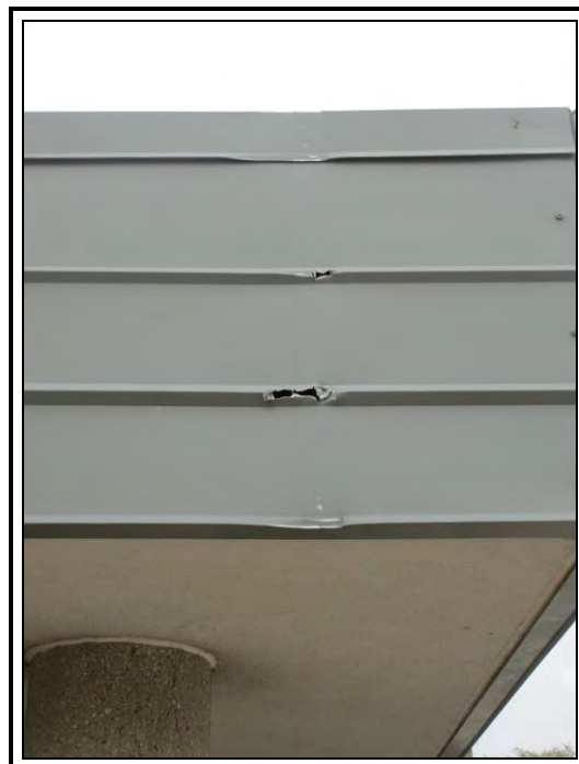
Photo 19: Roof Area 1: East Roof Edge: the existing sheet metal coping and fascia has been damaged.
